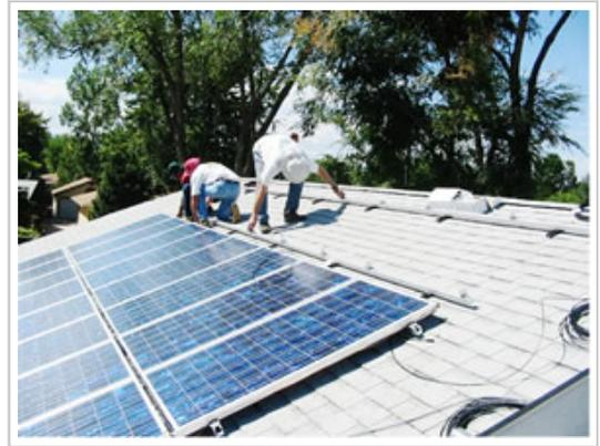
Crews installing solar thermal collectors and photo voltaic panels on the roof of a zero-energy house built for Habitat for Humanity. Photo by Pete Beverly
