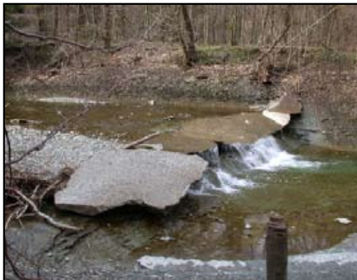
Sea Grant is helping to remove this concrete which will restore fish passage and natural flow to lower Fourmile Creek.
